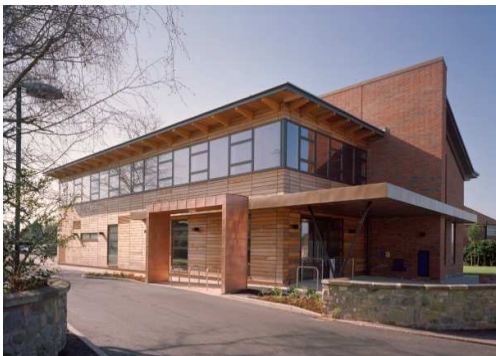
New Police station Market Drayton, Shropshire
